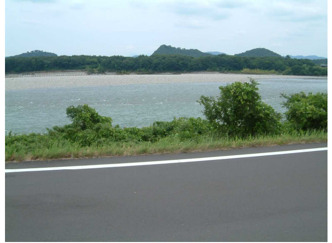
【Kiso River Embankment along Matsukura Castle Ruins】
